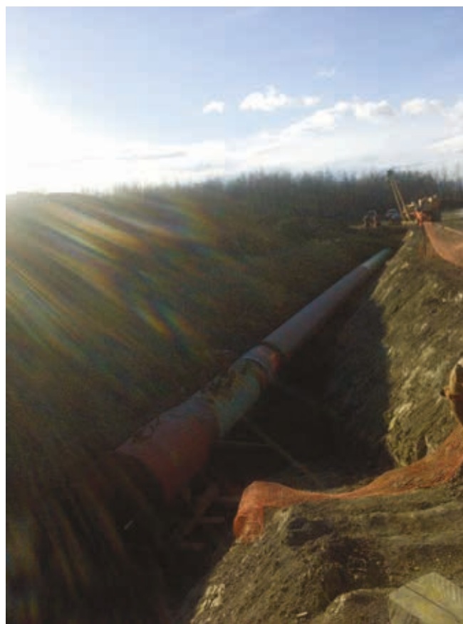
Figure 4. Site of a pressure test with exposed pipeline.
