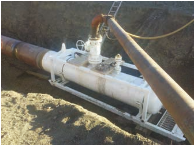
Figure 2. Pressure test in progress.
